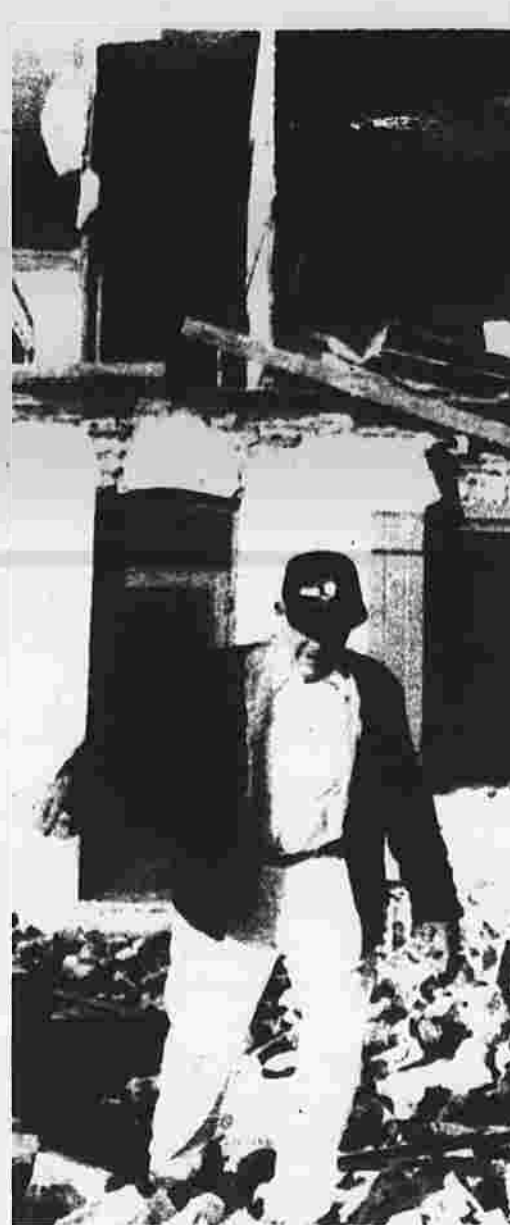
BUD O'NEILL INSPECTS RUBBLE that was once his house front wall
